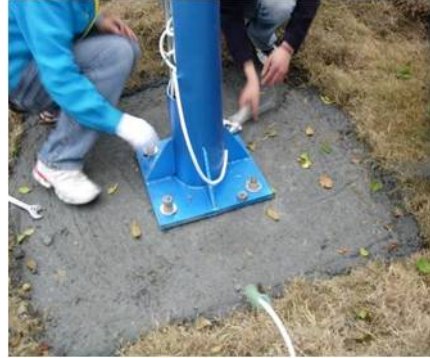
Place the washer and screw down the nuts on each bolt.
